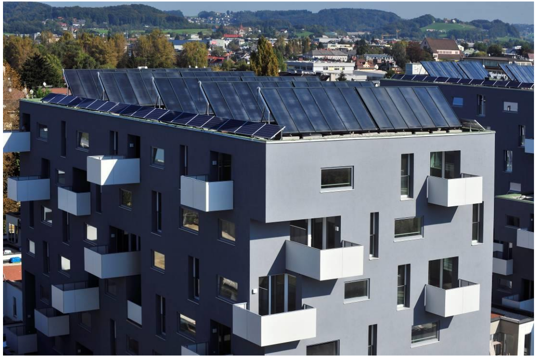
Fig.1.4 The effective use of solar energy PV and by thermal solar collectors. Fotohof Haus, Salzburg, Austria.
